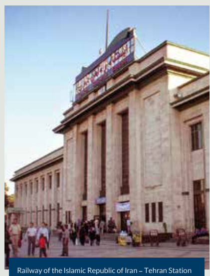
Railway of the Islamic Republic of Iran – Tehran Station İran İslam Cumhuriyeti Demiryolu – Tahran İstasyonu
